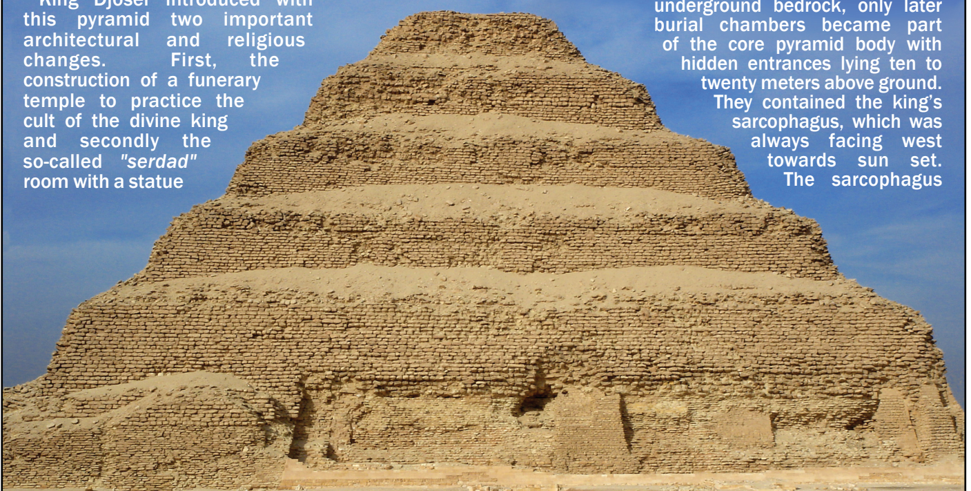
First pyramid erected as step pyramid with mud bricks for King Djoser 4,700 years ago
