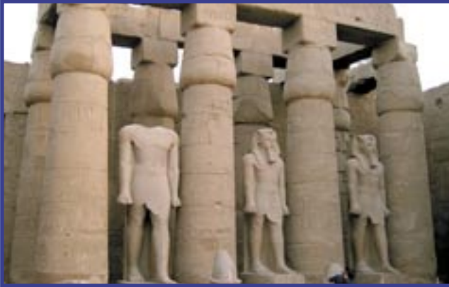
Corner view of double colonnaded courtyard built by Ramses II with 74 lotus bundle style columns supporting the missing roof with 7m high statues of the pharaoh.
