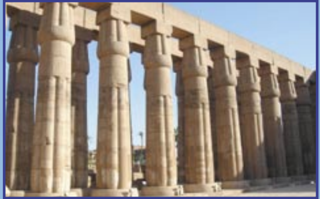
Second ceremonial tenemos measuring 52m by 46m surrounded by double row of papyrus bundle shaped colonnades with open inner area built by Amenhotep III.
